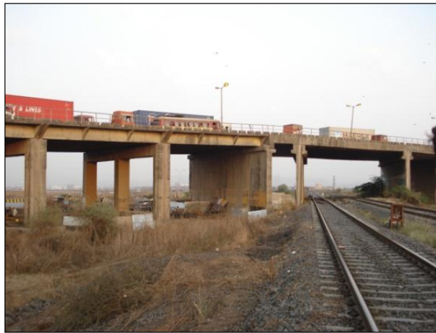
Figure 1. ROB ( Rail Over Bridge) at Karal Junction, JNPT
