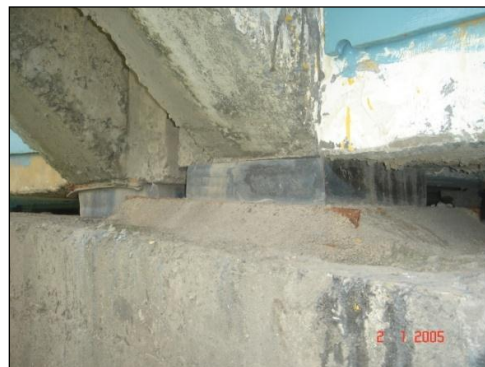
Fig. 4 Replacement of damaged Bearings with new
