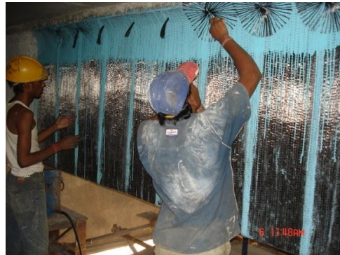
Figure 6. Enclosing the girders with Carbon Fiber Wrapping
