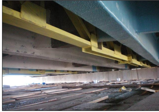
(a) Connection of Truss over Diaphragm Beam
